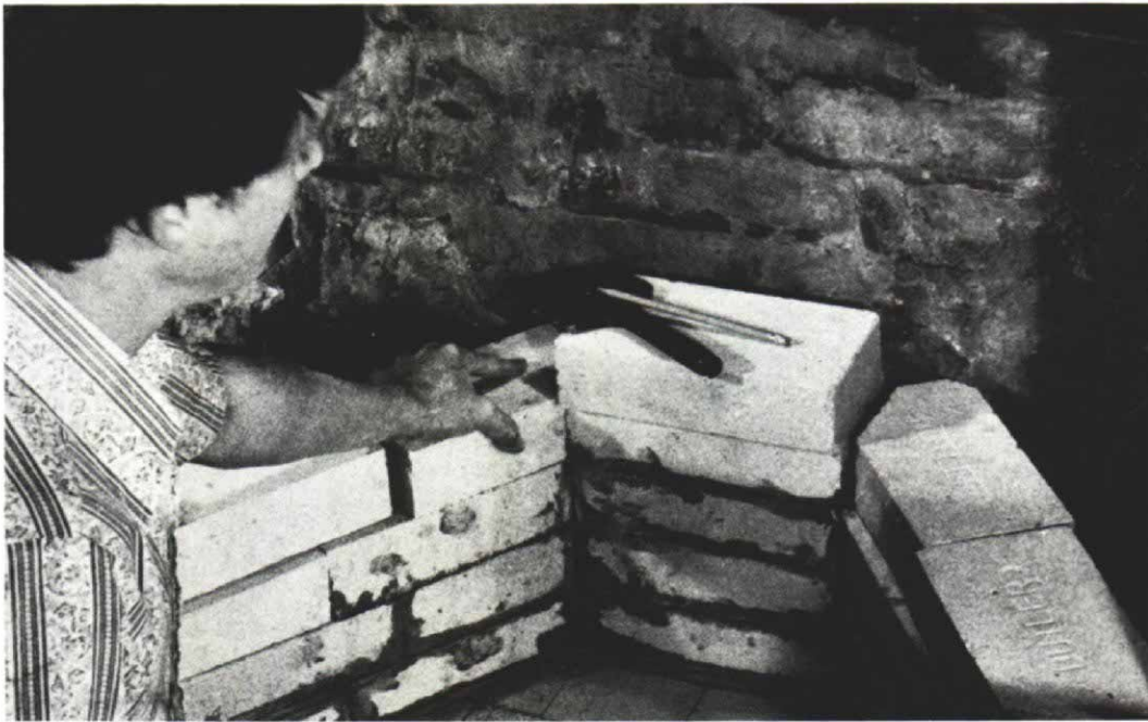
When the fireback is only one brick long, the most efficient way to butt coving and fireback is to cut the coving brick to fit along the fireback's header, left. When the fireback is longer, cut the coving brick to fit against fireback stretchers. Above, firebox is filled in behind with rubble and masonry. A fairly wet concrete mix will flow to the bottom.
