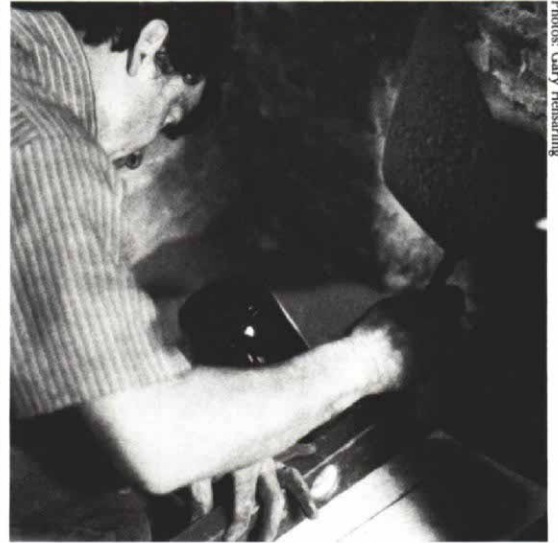
Fireboxes aren't structurally connected to the masonry of the chimney. You can often tear one out, as at left, by reaching up and tugging. Above, the underfire should be installed dry, without fireclay between the bricks. Be sure each brick is set level. (The bottle is covering an old gas line that will become a fresh-air intake.)
