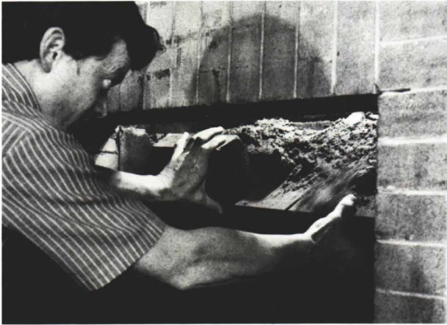
Fireboxes aren't structurally connected to the masonry of the chimney. You can often tear one out, as at left, by reaching up and tugging. Above, the underfire should be installed dry, without fireclay between the bricks. Be sure each brick is set level. (The bottle is covering an old gas line that will become a fresh-air intake.)
